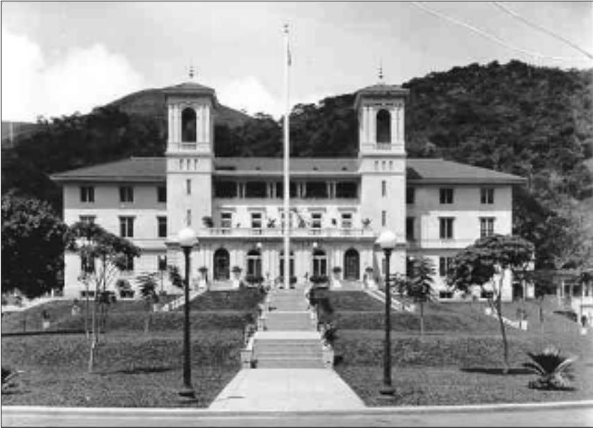
Afb. 4: Ancon Hospital in 1920
